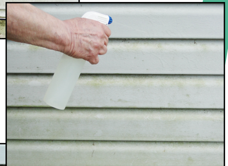
Spray Wayne Chlora Cling on mold.
