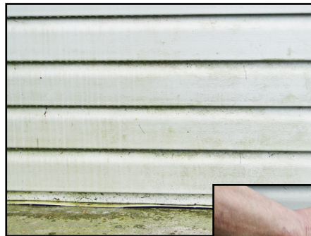
Mold stain on vinyl siding.
