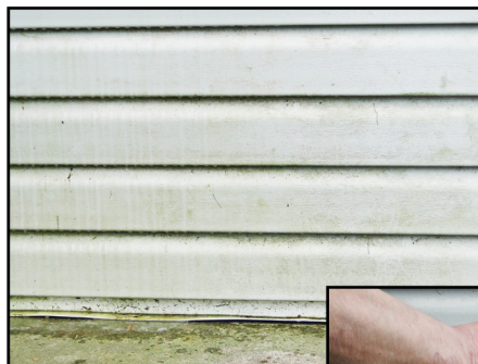
Mold stain on vinyl siding.
