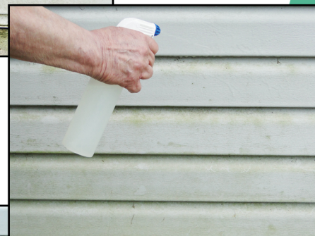
Spray Wayne Chlora Cling on mold.
